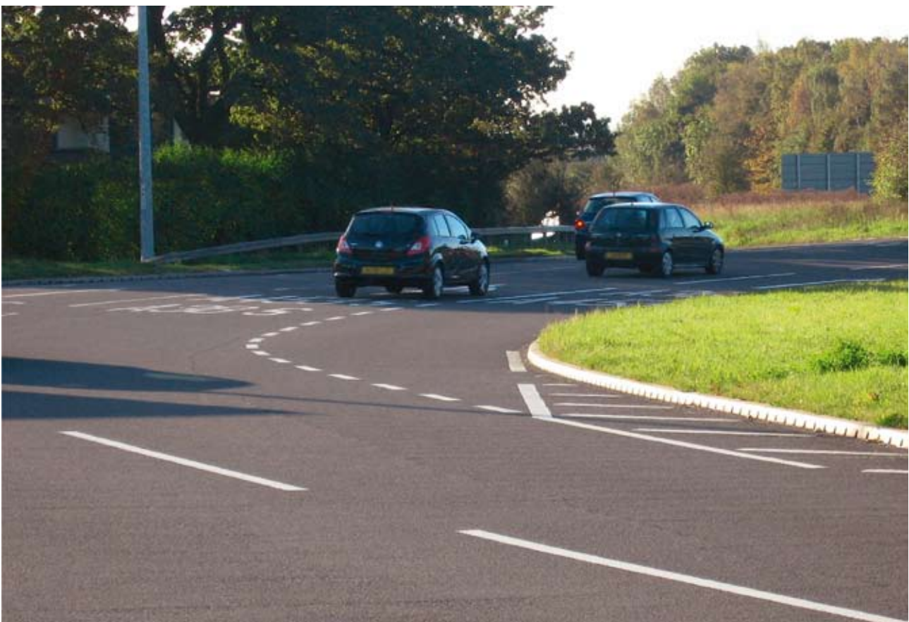
Figure 4.11 Spiral markings and hatching
