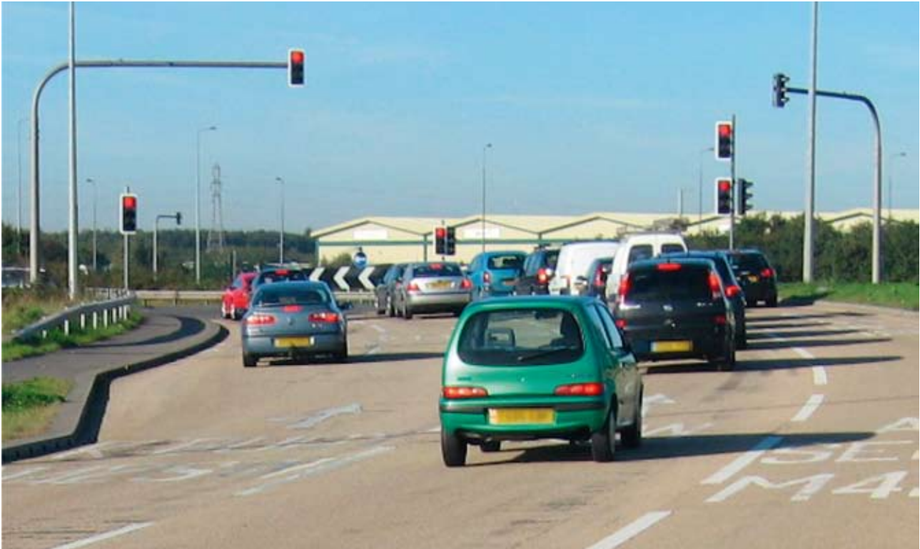
Figure 4.15 Mast arm signal – note location behind barrier
