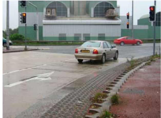
Figure 4.10 ‘Anti-pedestrian’ paving
